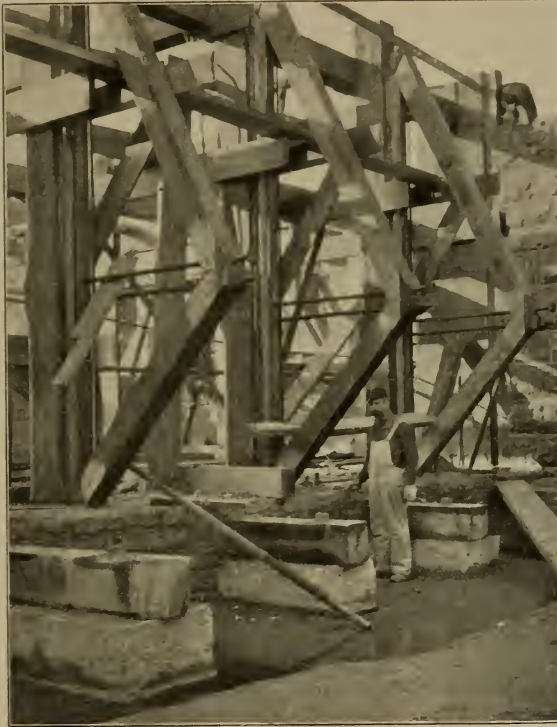
GATE POST BRACING—ROCKFORD GENERAL ELECTRIC CO.
